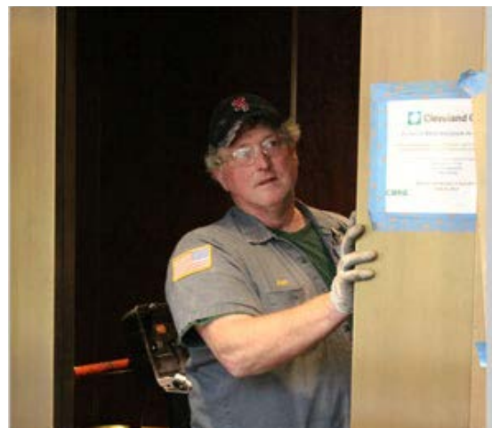
Cleveland Clinic is making energy efficiency improvements throughout our health system.
